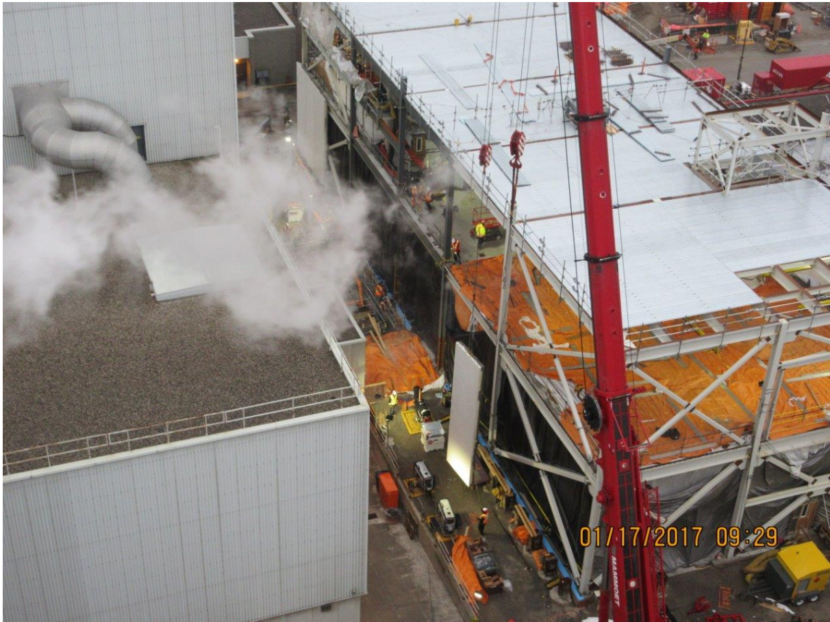
Figure 22 - Concrete Panel Installation on the East Side of the D2O Storage Building
