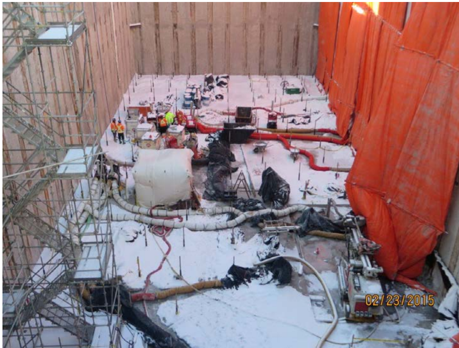
7 8 Figure 17 - Ground Heaters and Caisson Frost Protection Tarps
