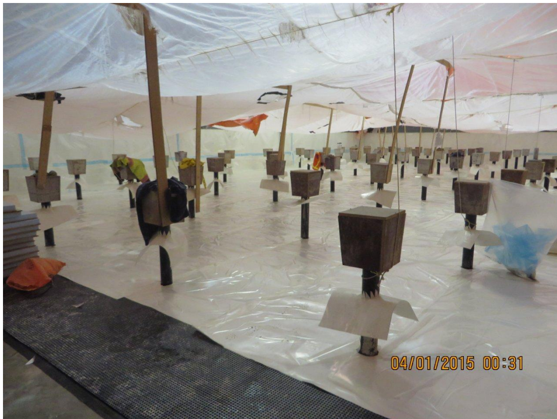
12 13 Figure 15 - Rock Anchor Sleeves with Wood Forms and Waterproof Membrane
