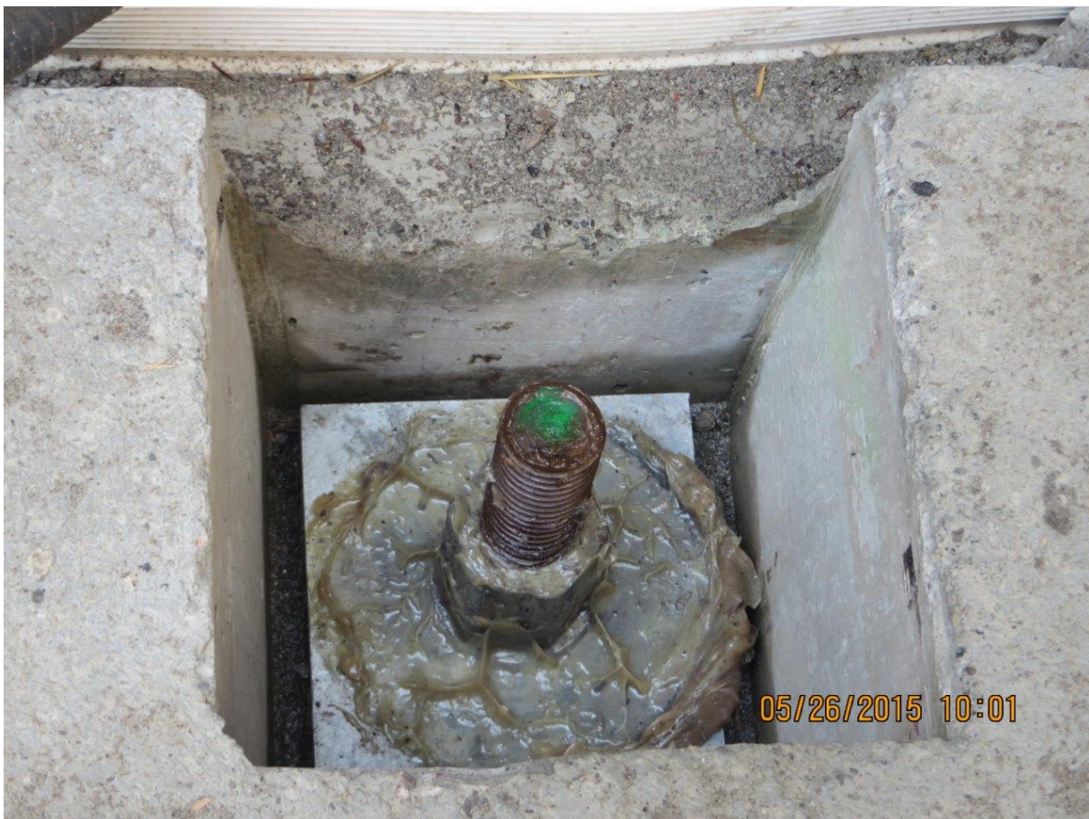
8 9 Figure 16 - Rock Anchor after Foundation Slab Pour with Nut, Washer and Steel 10 Bearing Plate
