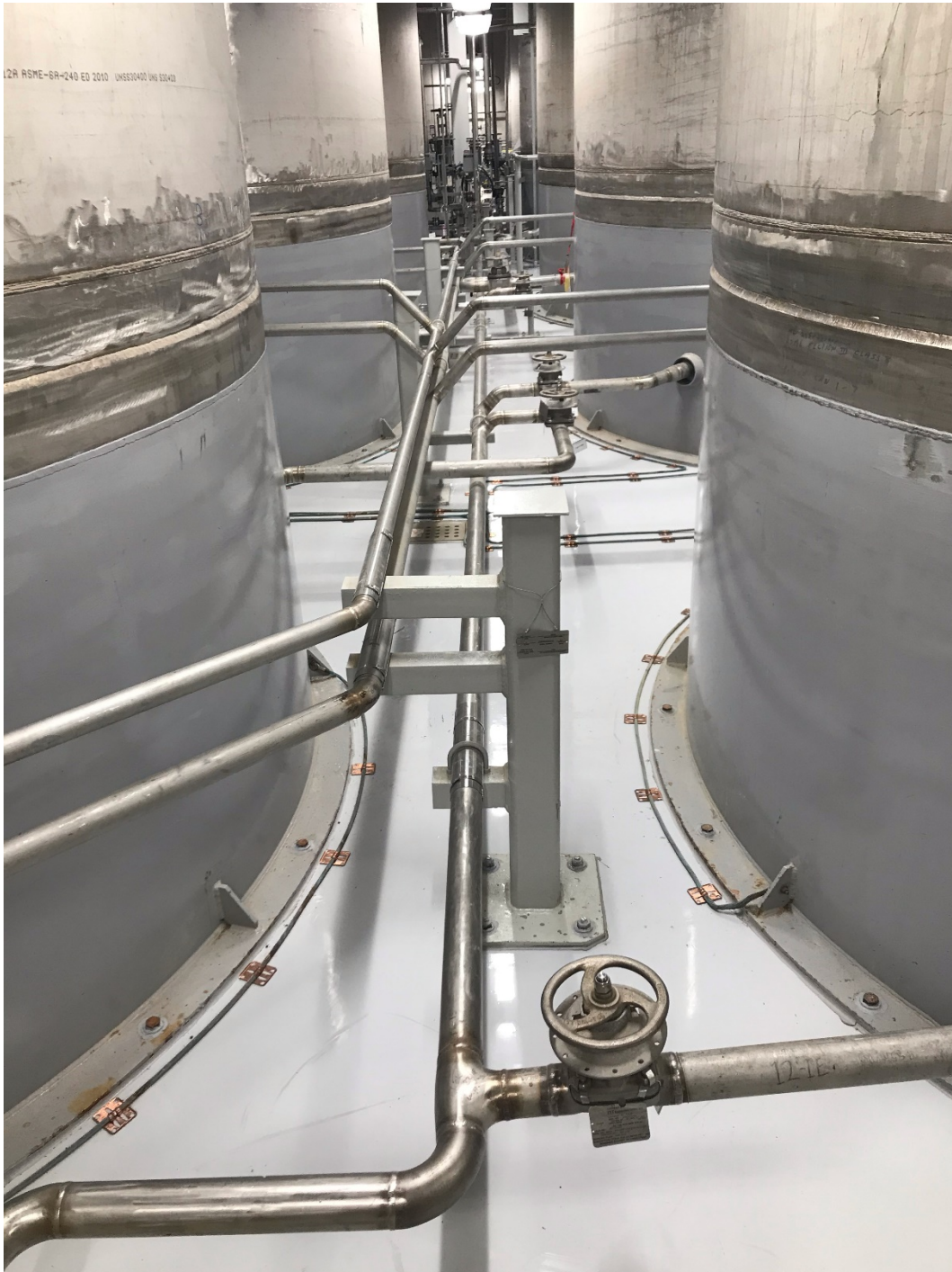
Figure 7 – Overhead View of Piping and Vales for the TRF Feed/Product Heavy Water Stream
