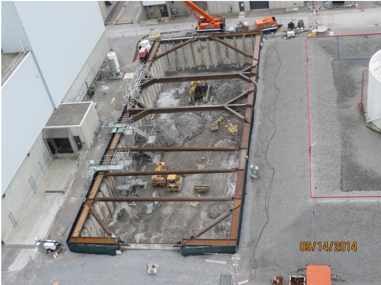
Figure 13 – Caisson Wall with Wailers, Struts, and Angle Braces during Excavation
