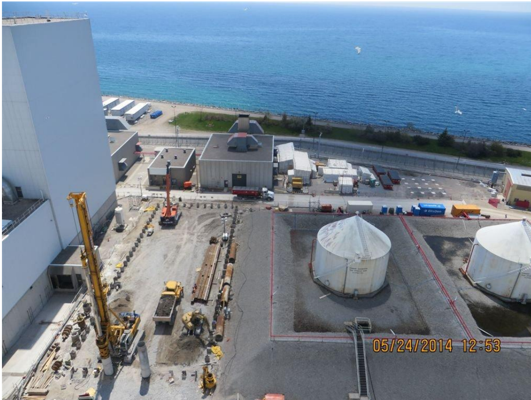
Figure 12 – Caisson Installation North Side of the Project
