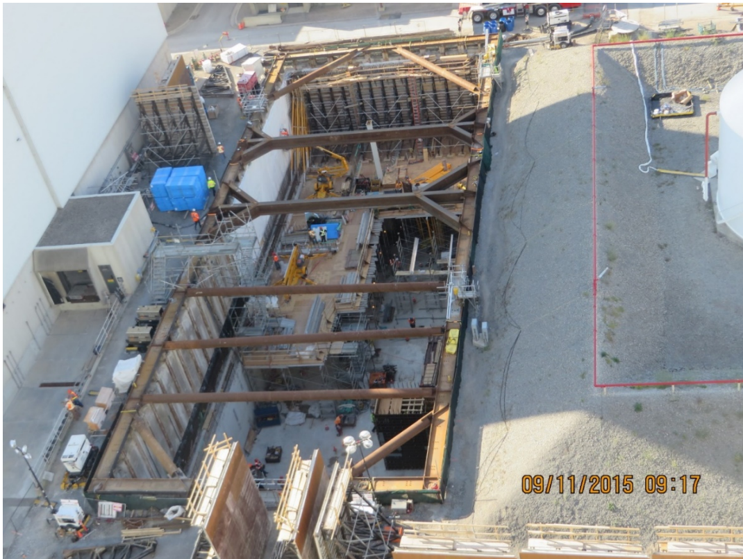
12 13 Figure 19 - Installation of the Top Half of the Seismic Dike South Wall
