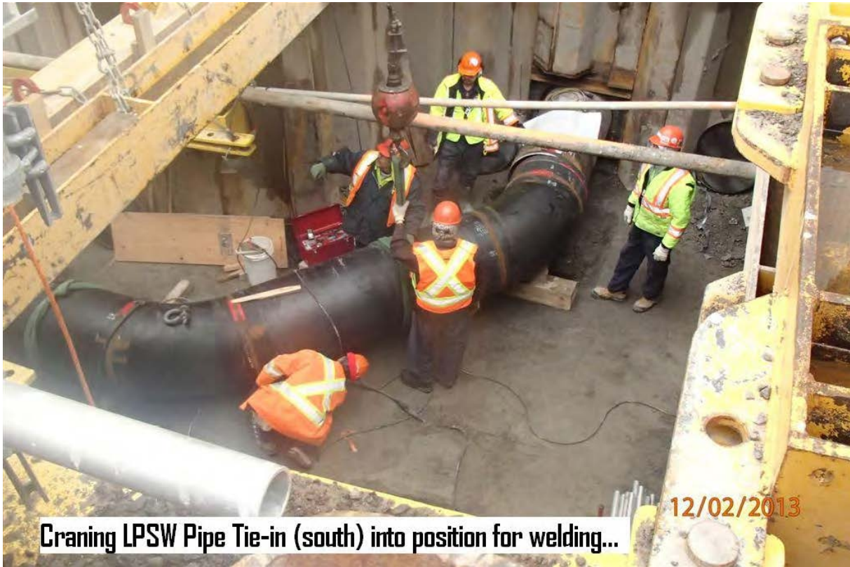
Figure 11 – Positioning an LPSW Pipe Angle
