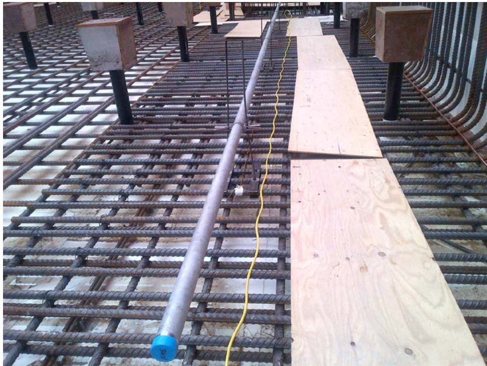
14 15 Figure 18 - Rock Anchor Sleeves with Forms, Rebar and Drainage Pipe Prior to 16 Foundation Slab Pour
