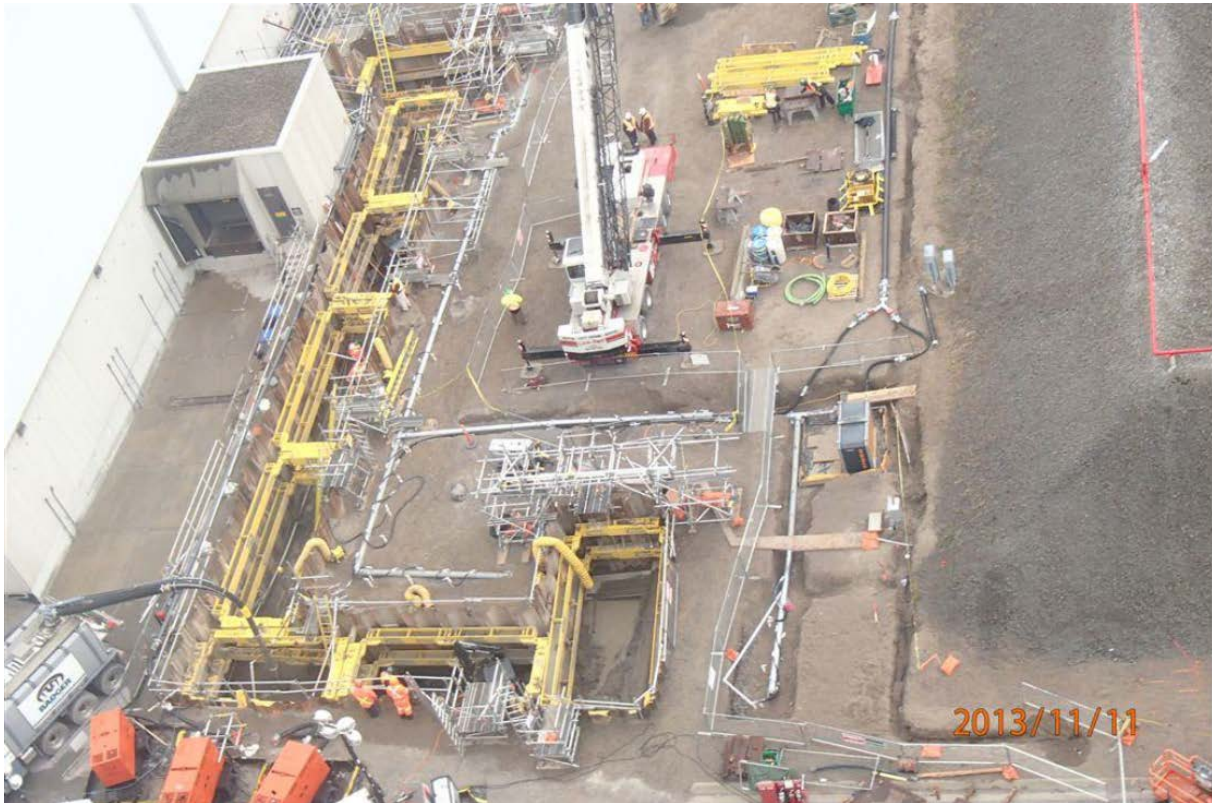
Figure 10 – LPSW Pipe Trench Prior to Installation of the New Pipe
