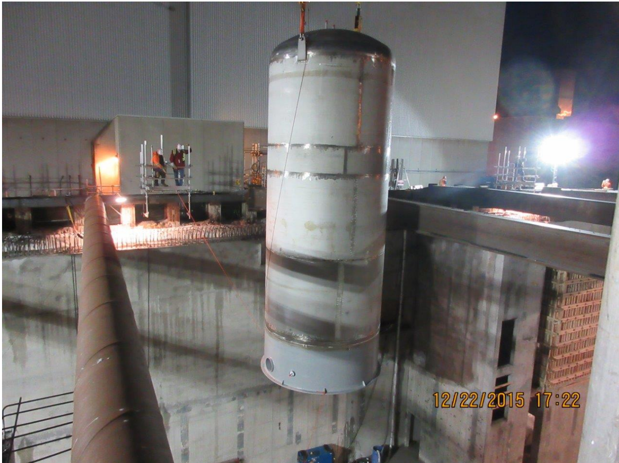
Figure 20 - Lowering the First D2O Storage Tank Into the Seismic Dike
